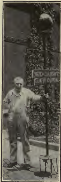
EMERGENCY LIGHT, USED AFTER ACCIDENTS TO FIXED STANDARDS
